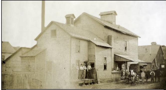
The Fire's Origin ... In Hoffman's Middleton Roller Mills
