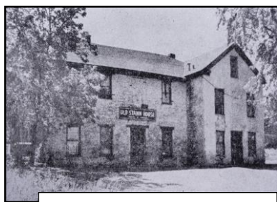
Early photo of Old Stamm House
